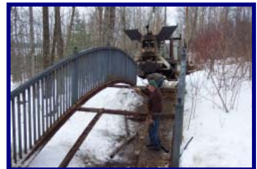
Ridgeline footbridge undergoes repairs.
