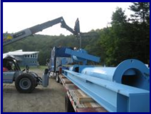
Unloading the drive terminal structure.
