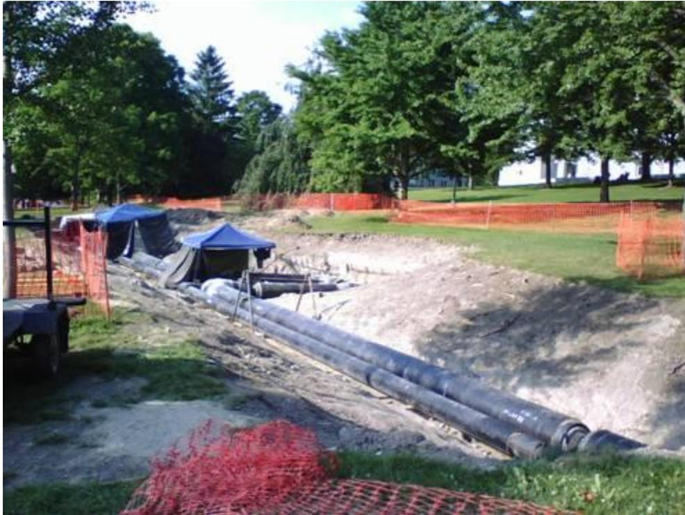
*Section of new underground steam pipe system installation – McCullough to Monroe Hall*
