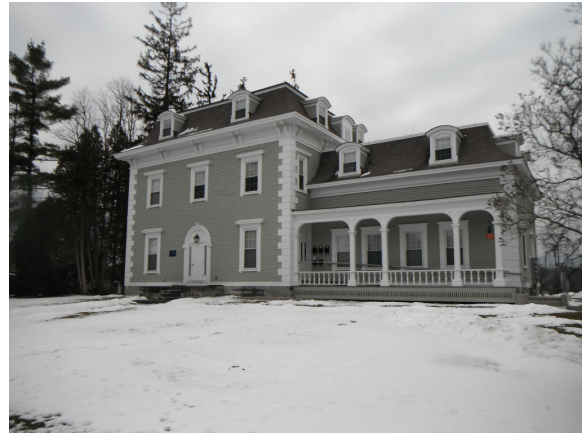
Fletcher House Following Renovation
