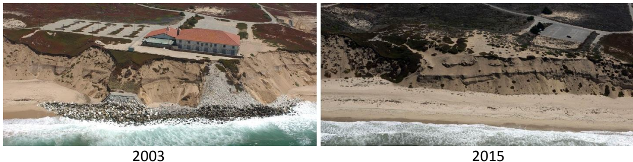
Figure 3: Stillwell Hall before and after removal of armoring and building in 2004
