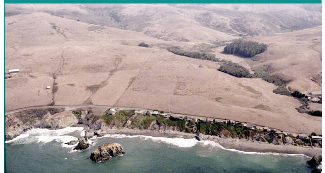
FIGURE 7: COASTAL INFRASTRUCTURE AT RISK
