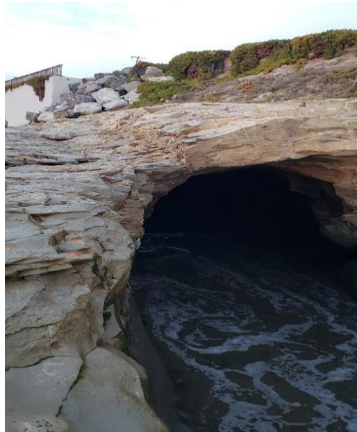
Figure 2-8 Cave Hazard near David Way in Zone 2.
