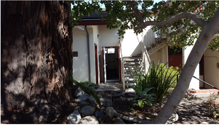
View of entrance to room B104. The entrance to room B104 is just past the redwood tree, nearest the stairwell leading to our upstairs breakout rooms.
