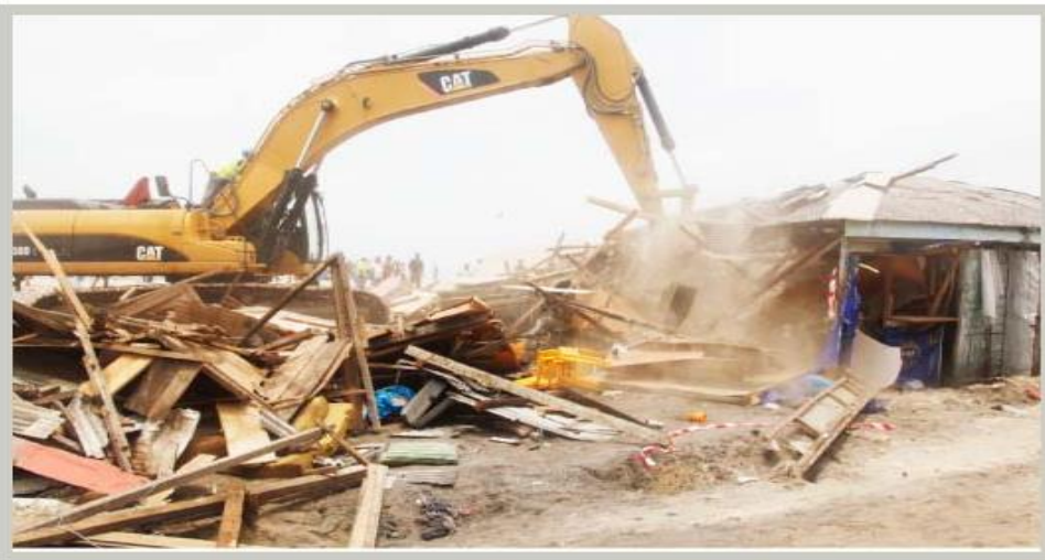
•Photo: Demolition at the beach , Photos: Kunle Ajayi
