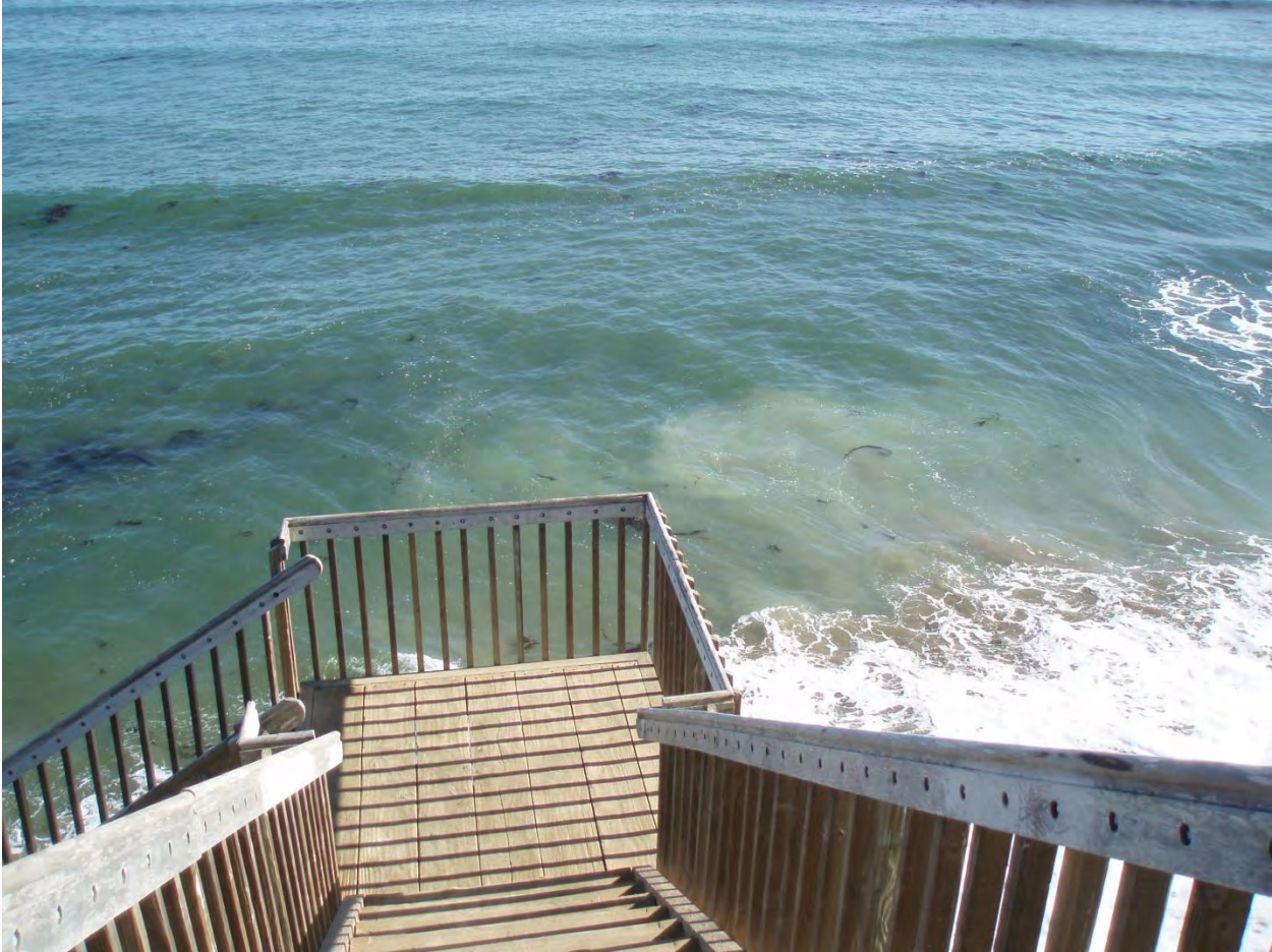
Beach Access Stairway:
