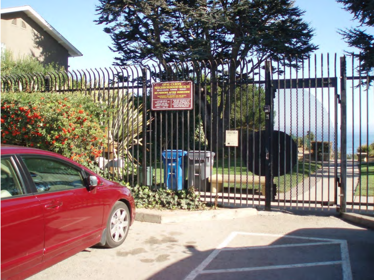
9-foot tall Wrought-Iron Fence/Gate:
