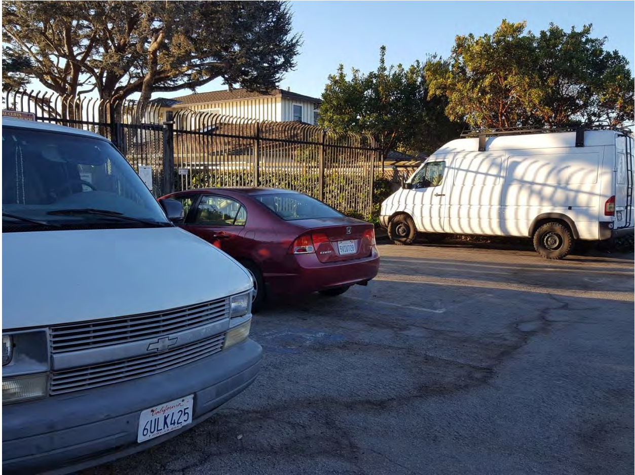
Fence/ Parking Area in 2018 (Note: No ADA Parking Signage and ADA striping is faded):
