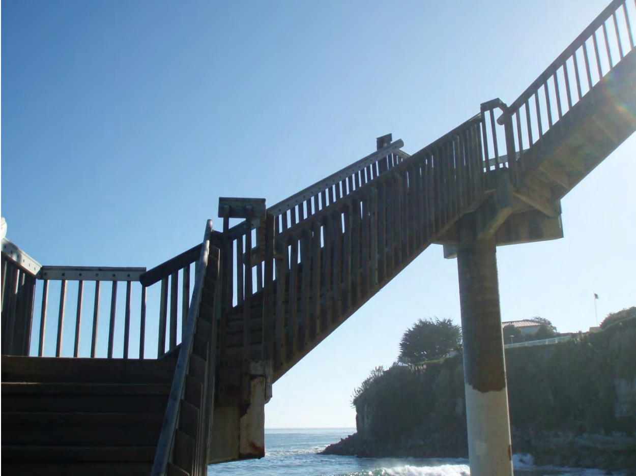
Beach Access Stairway:
