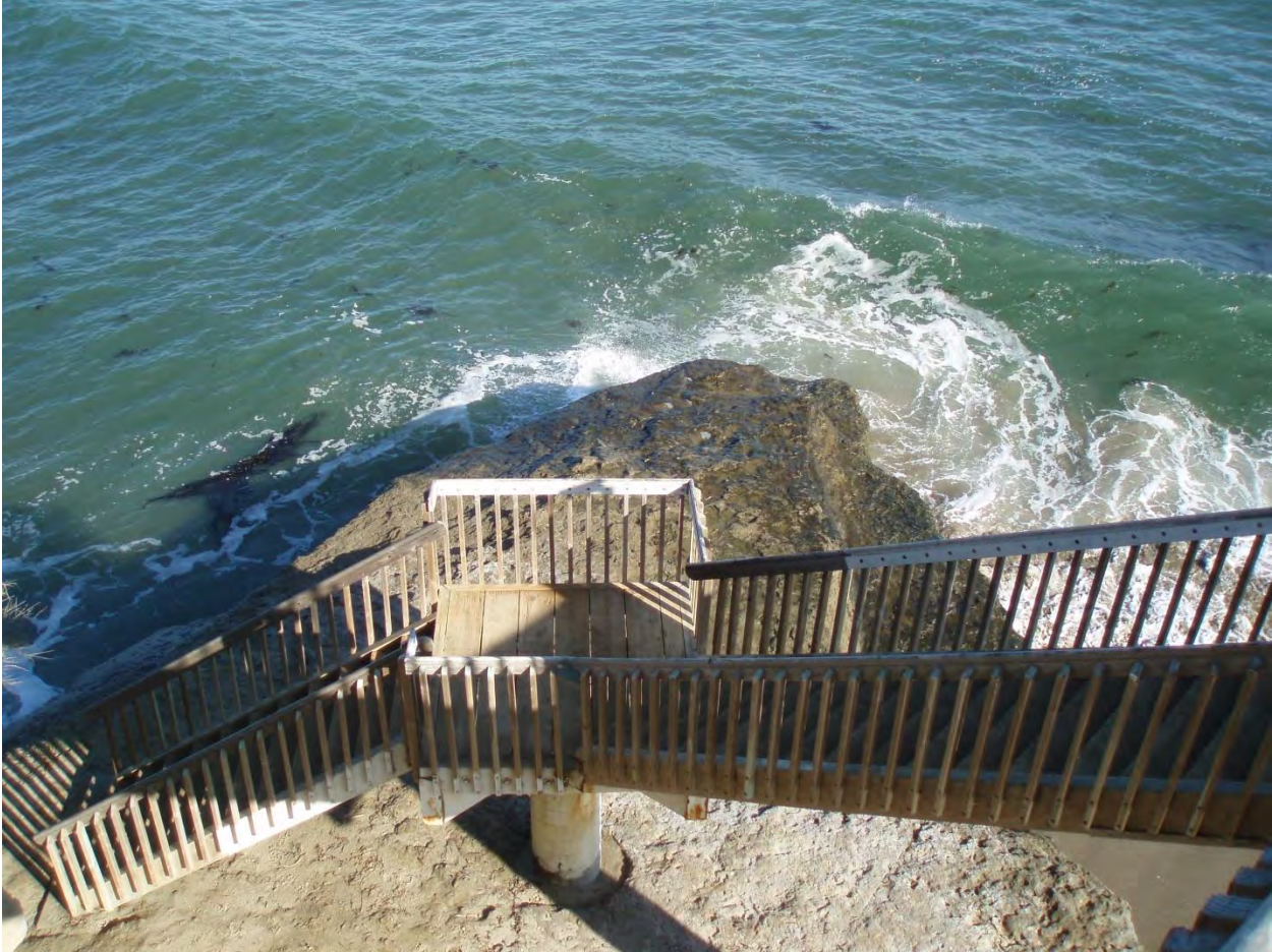
Beach Access Stairway:
