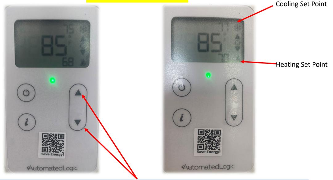
Press Up/Down Arrows for set point adjustment. Your range for cooling is 75-79. Your range for heating is 68-72.
