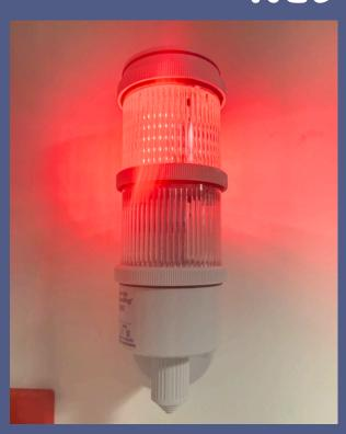
In labs with fume hoods, there is a red beacon that will illuminate if the room airflow is positive with respect to the hallway. Typically, the flow of air in labs with fume hoods moves from the hallway into the room, thus making the room negative to the hallway.
