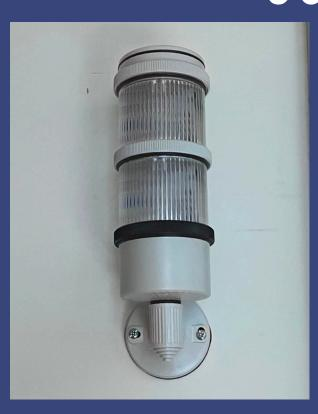
When the amber beacon is OFF, the room is in occupied mode.
