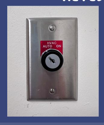
Some specialized labs now have a keyed switched for maintaining 24/7 occupied mode. This mode is only to be used when required for experiments needing consistent temperature/ventilation.
