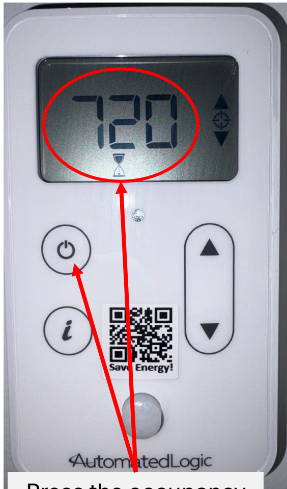
Press the occupancy button once to show the minutes the room will be occupied for temperature control.
