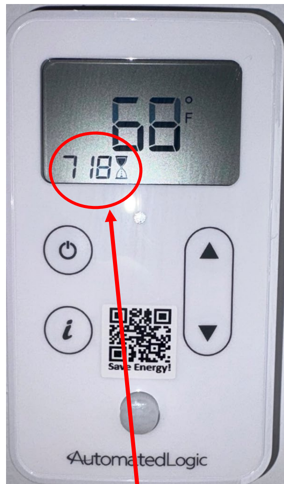
Pressing the button twice will cycle the timer to zero. Pressing once at any time, will reset to 720 minutes (12-hours).
