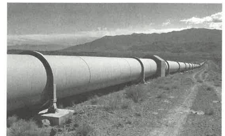
Figure 1-7 The Owens River is diverted through a large pipe to Los Angeles. Courtesy of Eric and Avery Wilmanns.
