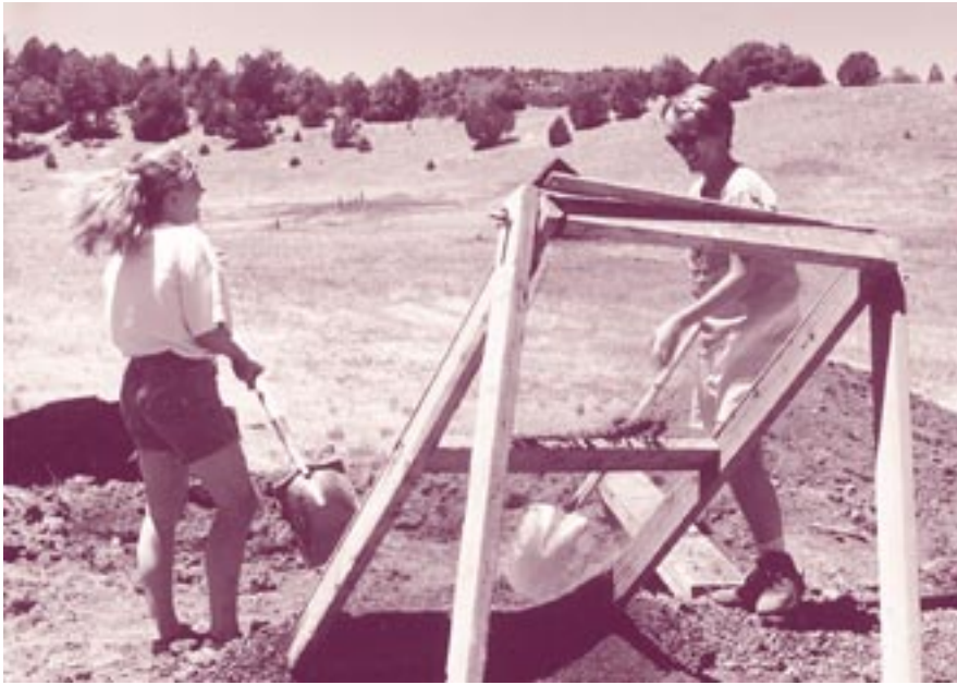
Bread Loaf students Melissa McKay and Christian Leahey sifting earth to make building materials for the Church at Cañoncito/La Cueva
