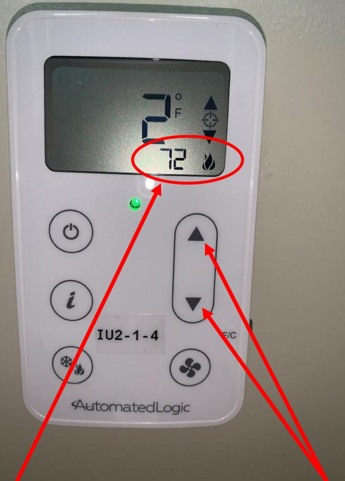
To adjust the set point for your space, first push the up or down button once. The current set point will be shown. Flame indicates heating and its set for 72. The green light indicates these are occupied set points.
