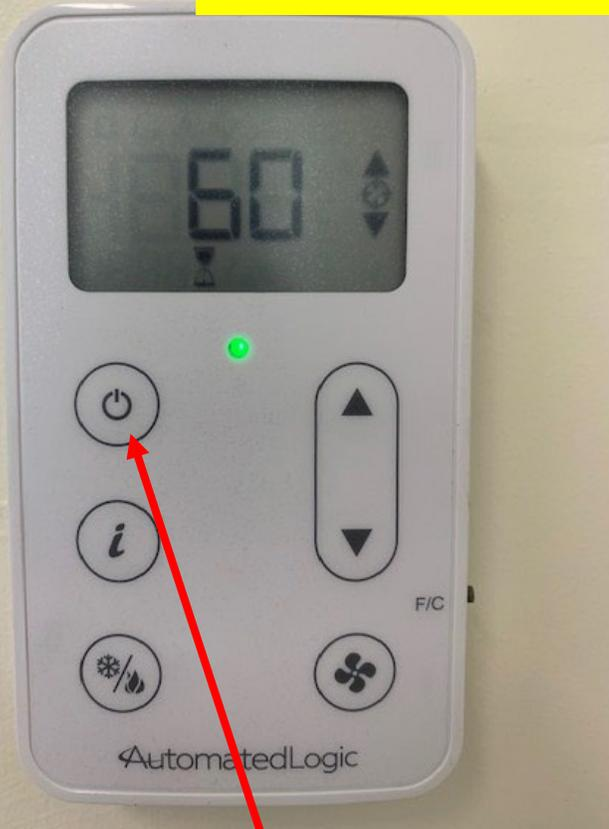
If you want to stop occupied mode, push a second time and "0" will show, which puts the time to zero minutes and the system will revert to unoccupied mode.
