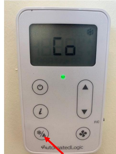
Push the button a second time and “cool on” will scroll across the screen. Only push the button twice, and then leave it alone. Once the occupancy light goes out (which is 30 minutes of the space being unoccupied) the system shuts off the cooling.
