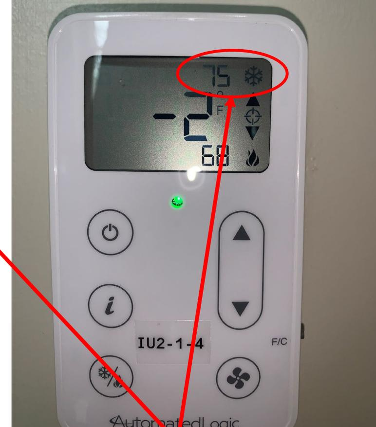
Notice the other pictures were missing the cooling set point. Those units had not been put in cooling mode. Once in cooling mode, the heating and cooling set points will show. (Default for cooling is 77)
