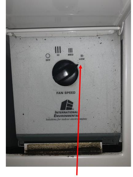
Low is a good position to leave the fan switch. You can play around with higher settings, but if the fan runs too hard, it can blow colder air than desired.
