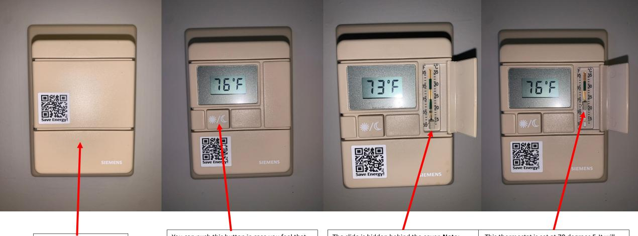
This thermostat is in a common space and has no slide adjustment. Set points are 75 for cooling and 70 for heating.
