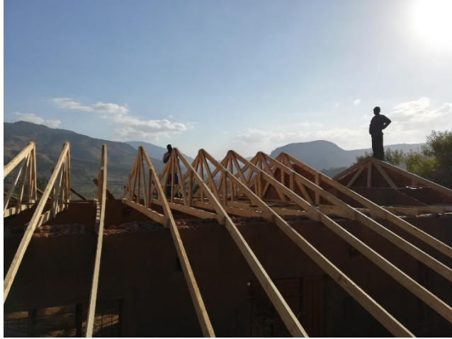
(The Chikukwa library under construction)
